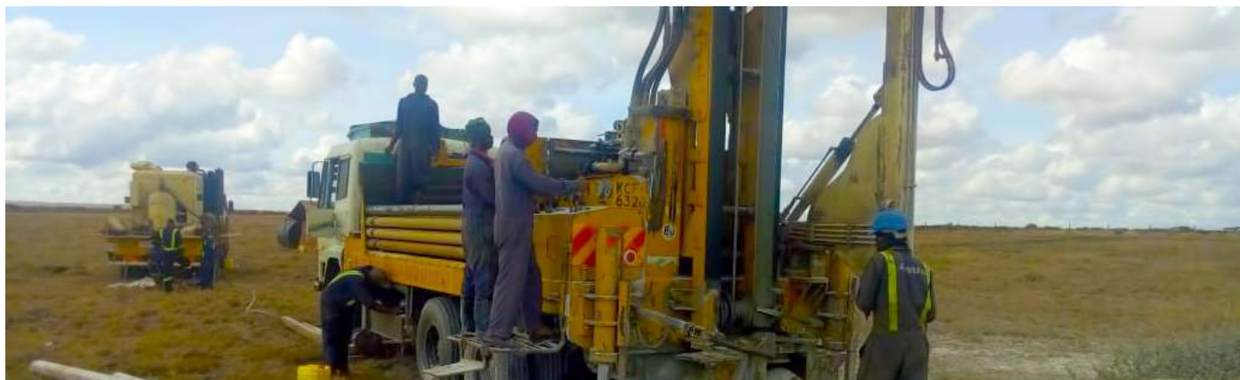
Borehole drilling at The Haven Konza project
