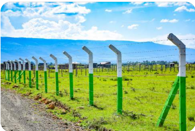
Springfield - Nakuru - Installation of an all-round perimeter fence with concrete poles complete
